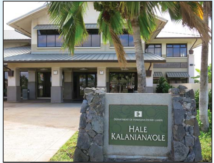
DHHL secured new headquarters of 50,000 sf in Kapolei and adjacent to a number of their strategic parcels
